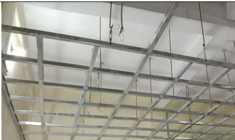
Sample Frame Structure for False ceiling
